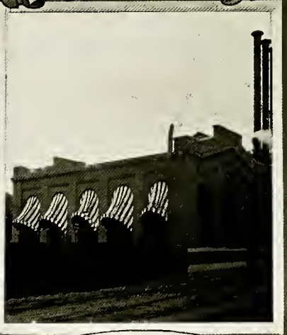
ADDITION TO POWER PLANT
